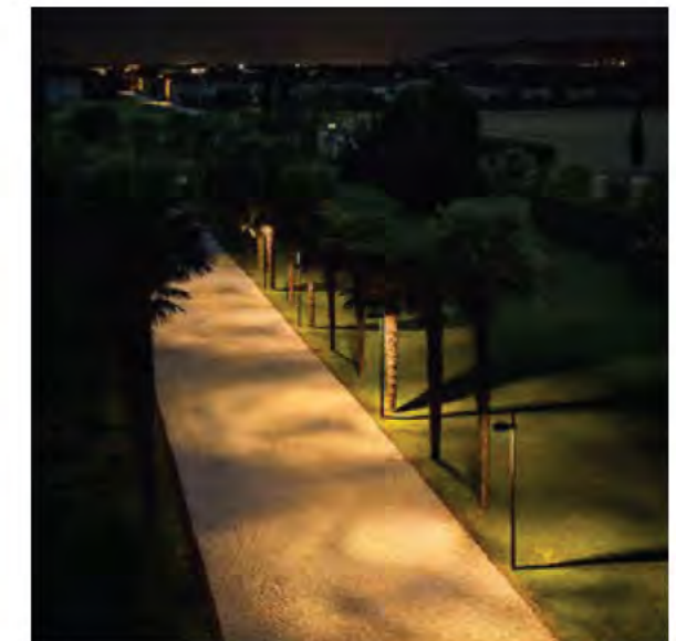
Light columns with a directional lumiere to prevent light spill
