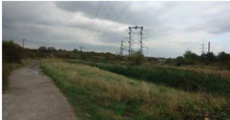
Wider pathway alongside pylons (DS1)
