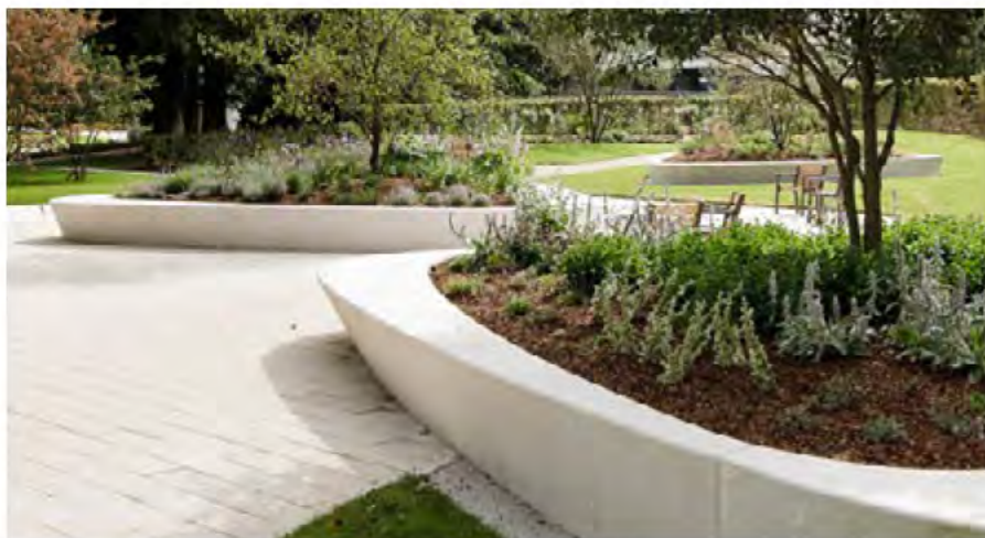
Seat walls defining planters
