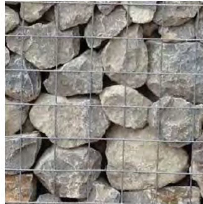
Kentish ragstone gabions can be utilised in marsh areas, potentially to form flood embankment edges or sea walls
