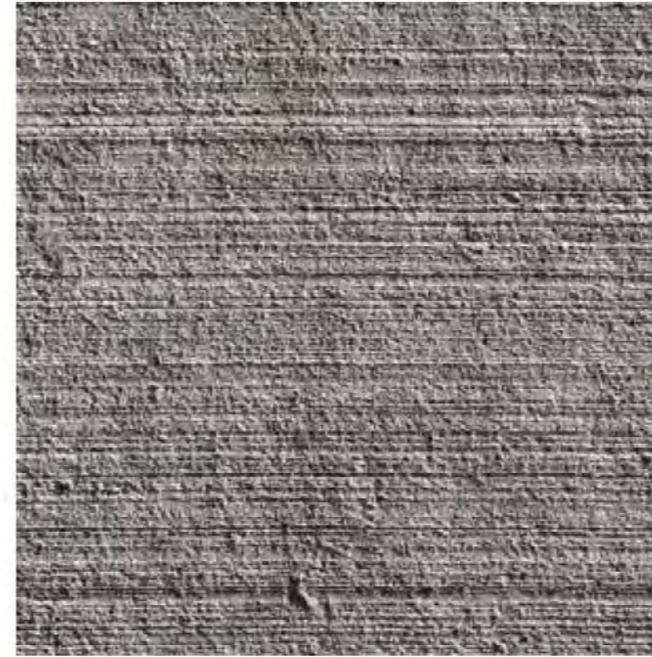
Concrete walls using pulverised fuel ash to cut down on cement
