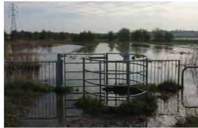
Surface water flooding issues in the marshes make some PROWs inaccessible
