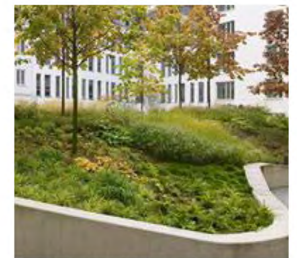
Raised planters define the edges of the plaza space
