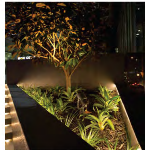
Concealed LED fixtures in planter minimising uplighting
